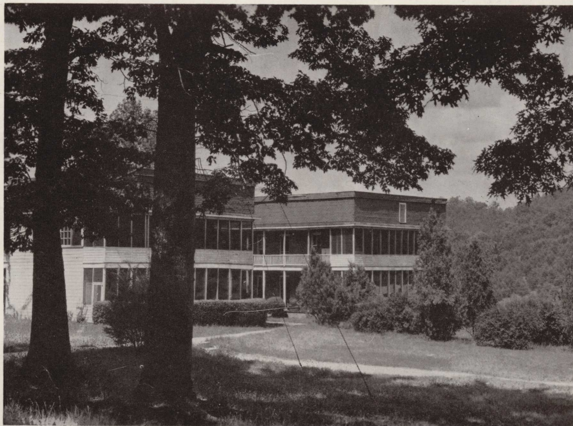
Right: The well with the Chapel in the background. Below: Hamby Hall.
