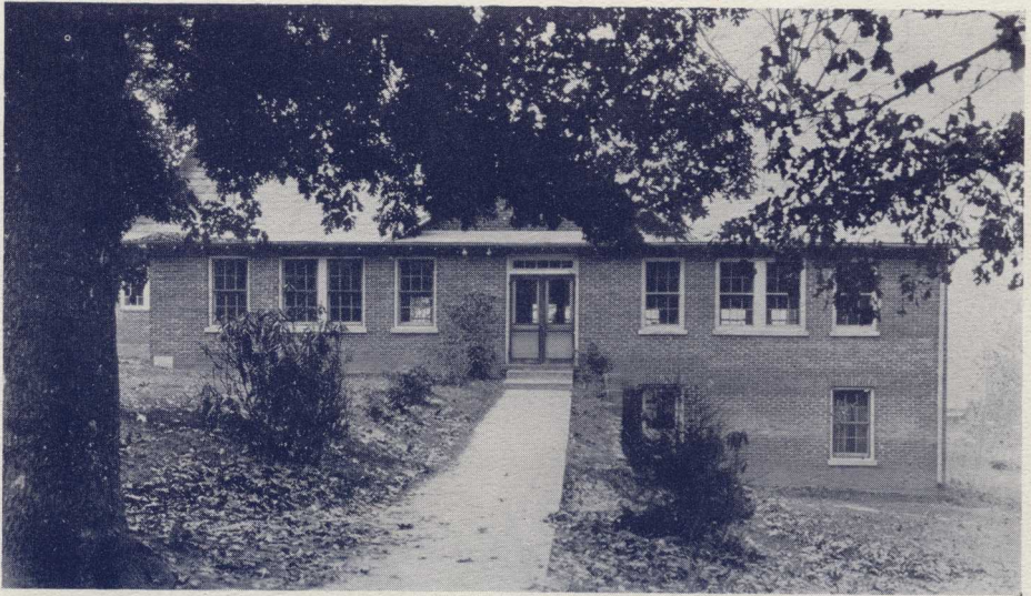
Library and Office Building
