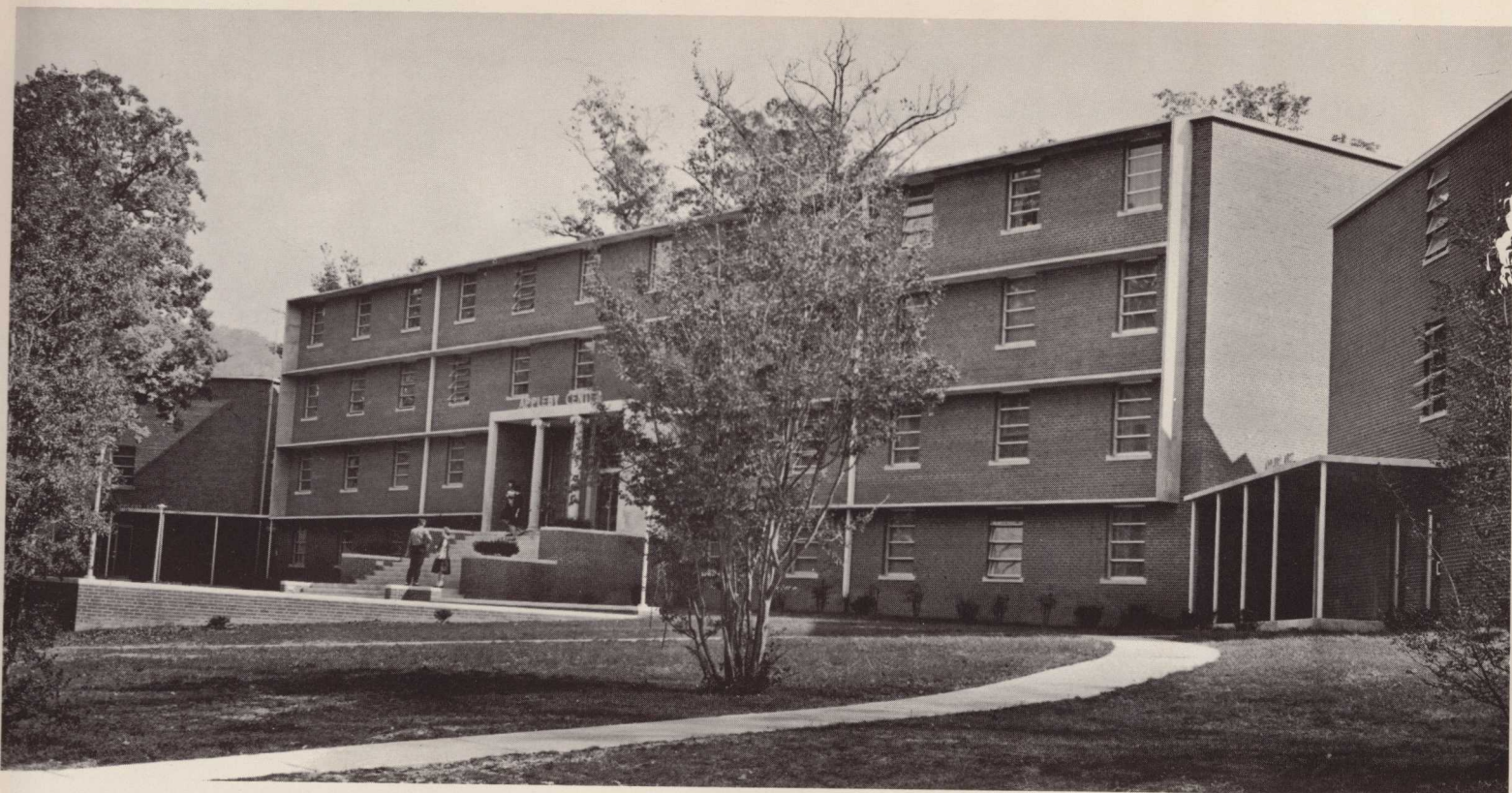
The new Appleby Center for girls nestles at the foot of the mountain. The two wings are connected by a central four-story building which houses over a hundred girls.
