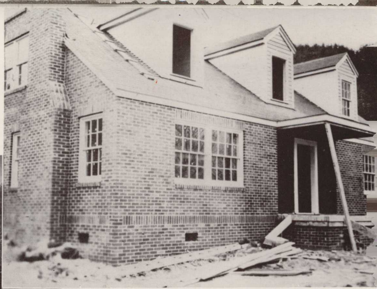
The new $10,000 parsonage under construction.
