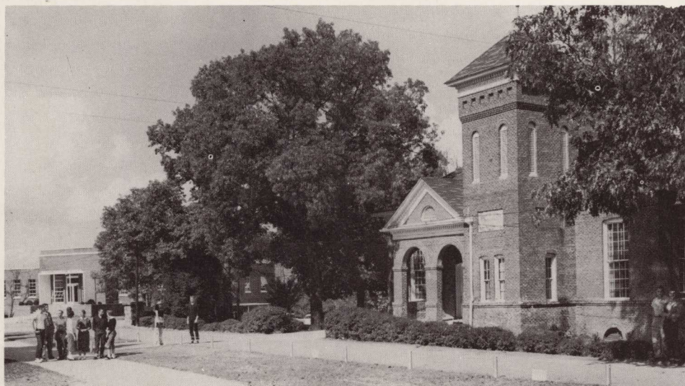
SUSAN B. HARRIS CHAPEL AND PRUITT-BARRETT BUILDING
